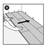
Once you have laid 1-2 rows of tiles the floor should be fairly rigid. Now you can slide it slightly away from the far wall, insert 8mm spacers and then push the tiles back into position.
