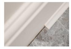
Expansion gaps must be allowed at the perimeter of the room and around all fixed objects. For rooms up to 10m length, this gap should be at least 5mm and can be concealed underneath skirting boards or with a beading. We recommend 10mm when rooms are larger than 10m in length, and also where direct
