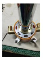
14. Slide the chrome cover plate down and install the handset.
