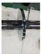
4. Wrap PTFE tape on the supplied elbows and install elbows into the easy-plumb box
