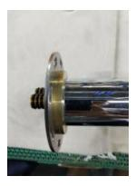
12. Fit the copper pipe from the standpipe to the easy-box connector, ensuring hot and cold align correctly relating to lever control
