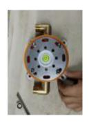
5. Set the easy-plumb box into the recess in the floor and ensure it is level using the spirit level provided
